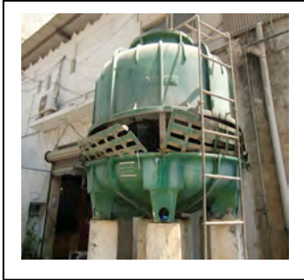
Damage of air in let louver
