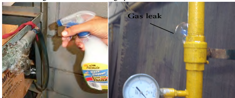
Figure 2-4 Spraying soap water Figure 2-5 Soap bubbles of leaked joint
