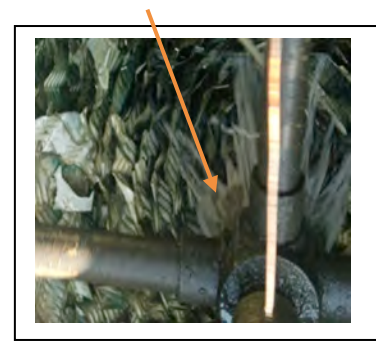
Leakage from shower head
