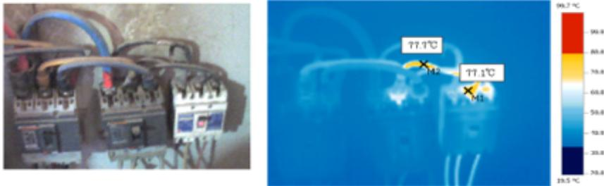
Maximum allowable temperature for PVC cable is 70degC. (Fast Cables Ltd.)
