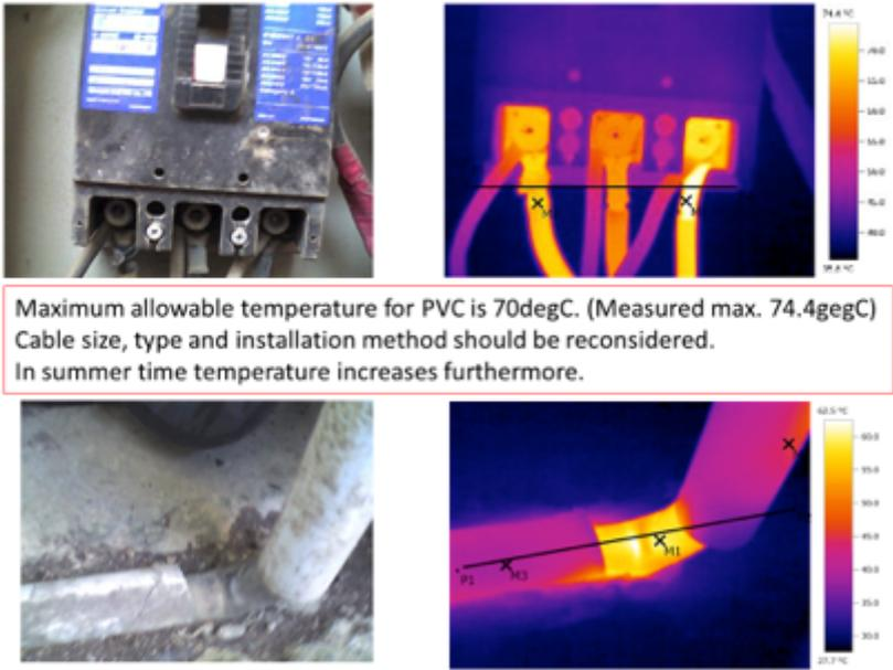
**Results:** Additional cable was installed for increasing cable size (double cable system).
