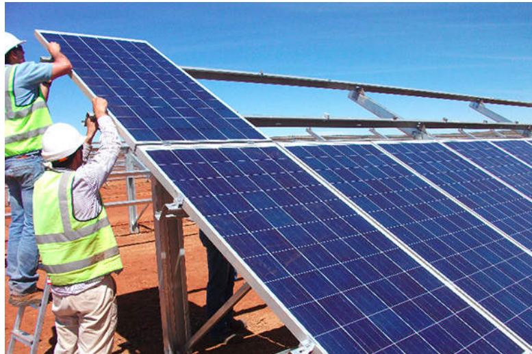
Figure 15: Mounting of Panels on Foundation
