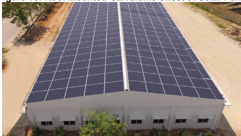
Figure 18: Roof Mounted Galvalume Sheet of Solar Panel
