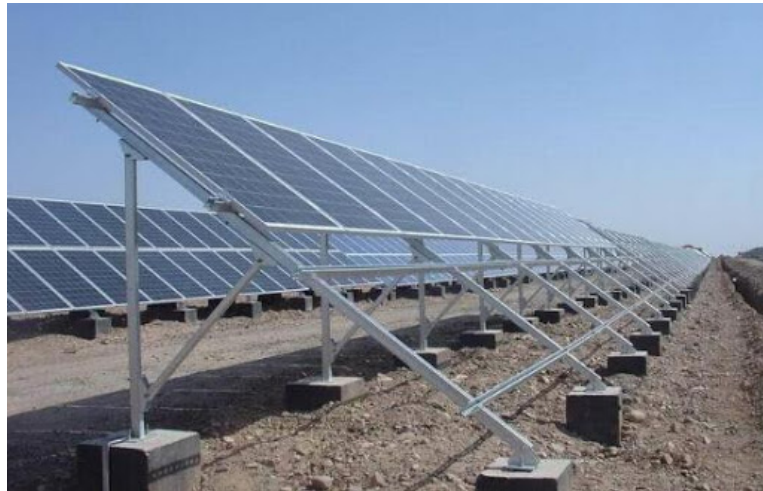
Figure 14: Civil Foundation of Solar Panel
