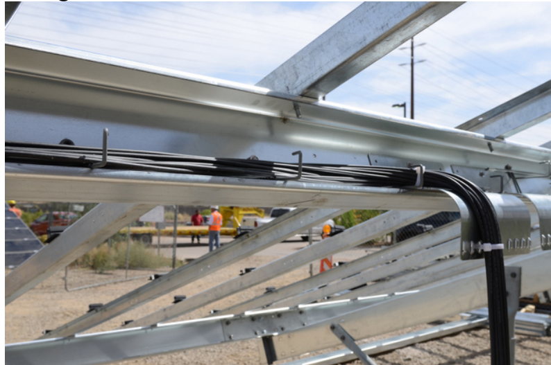
Figure 19: Wires Connected to the Solar Panel
