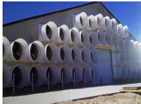
Figure 3: A typical ventilation system in ECH system
