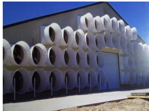
Figure 3: A typical ventilation system in ECH system
