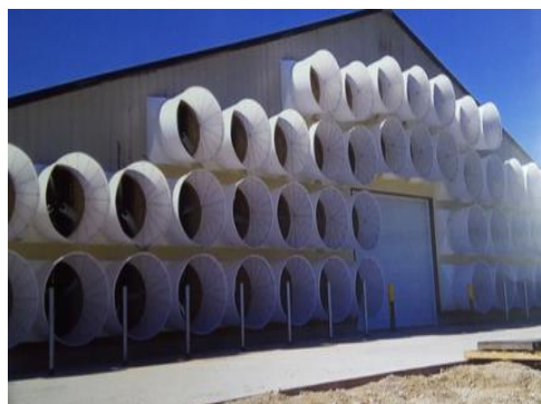
Figure 3: A typical ventilation system in ECH system
