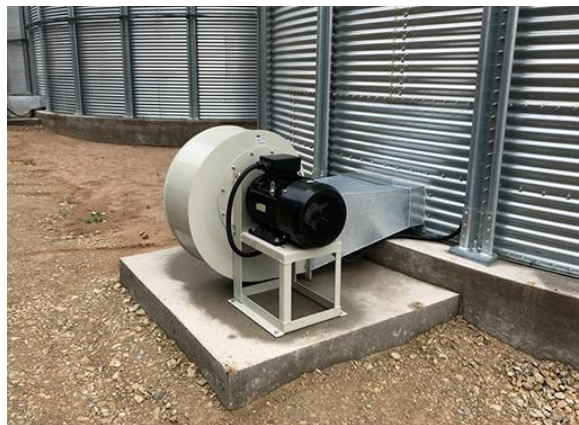
Figure 10: Installed Aeration System
